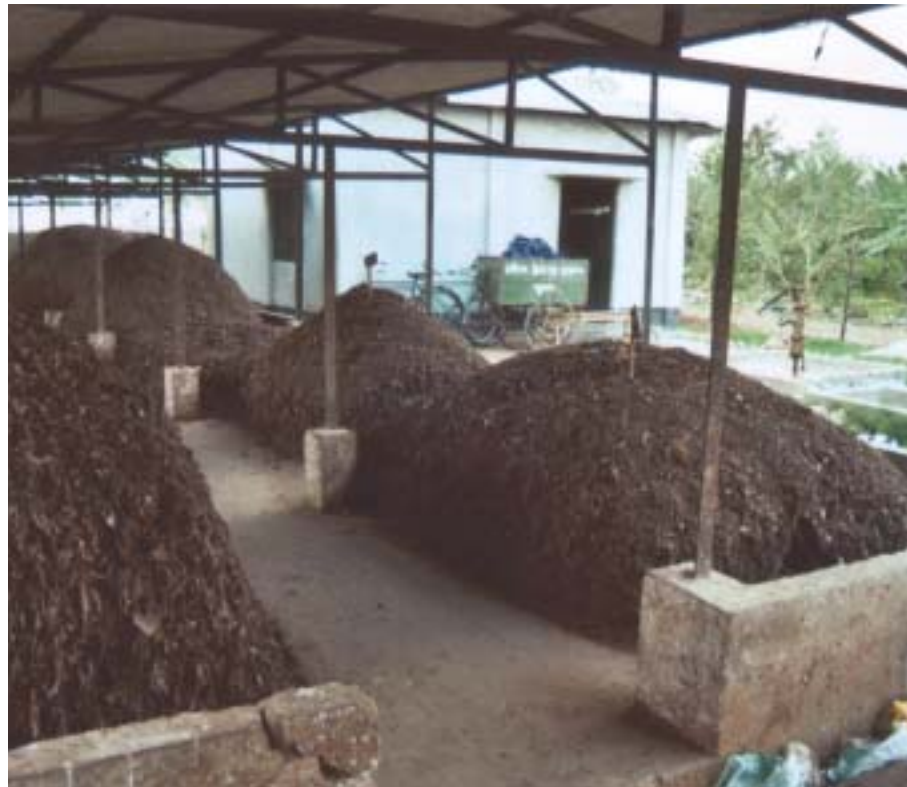
Medium-scale windrow composting plant.
